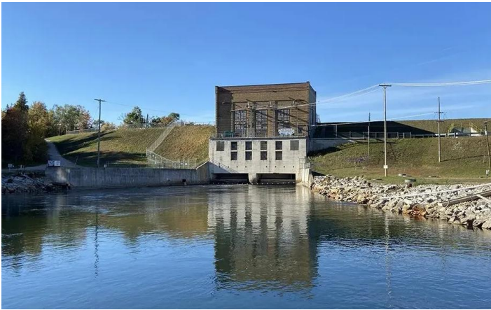
Alcona Dam, pictured here. (Kelly House/Bridge Michigan)
